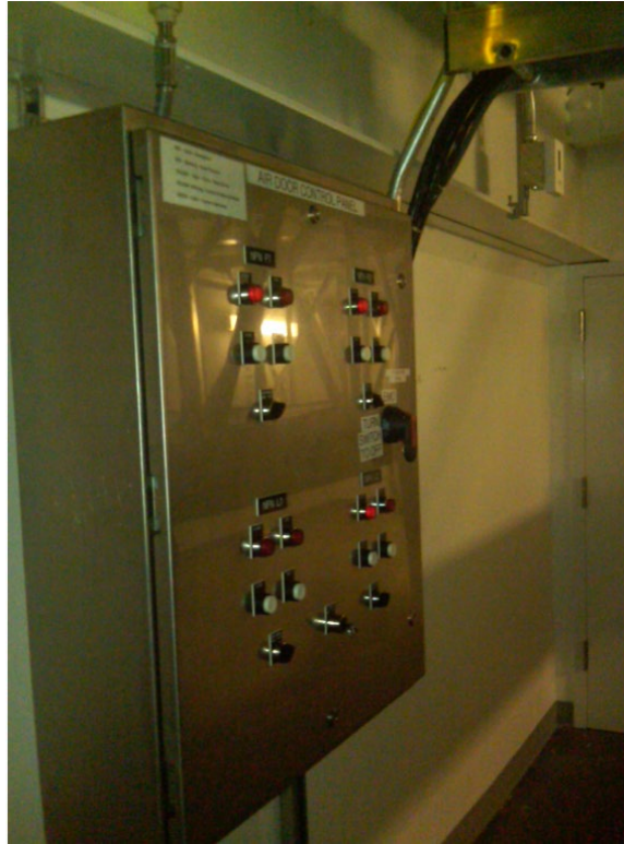
Figure 2. Air Door Controller
