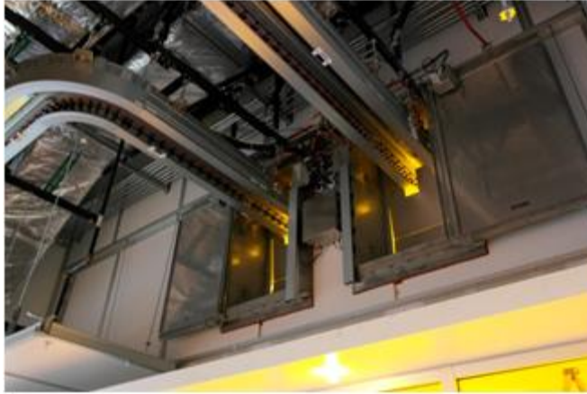
Figure 5. Fire Doors in NFX Link Area
